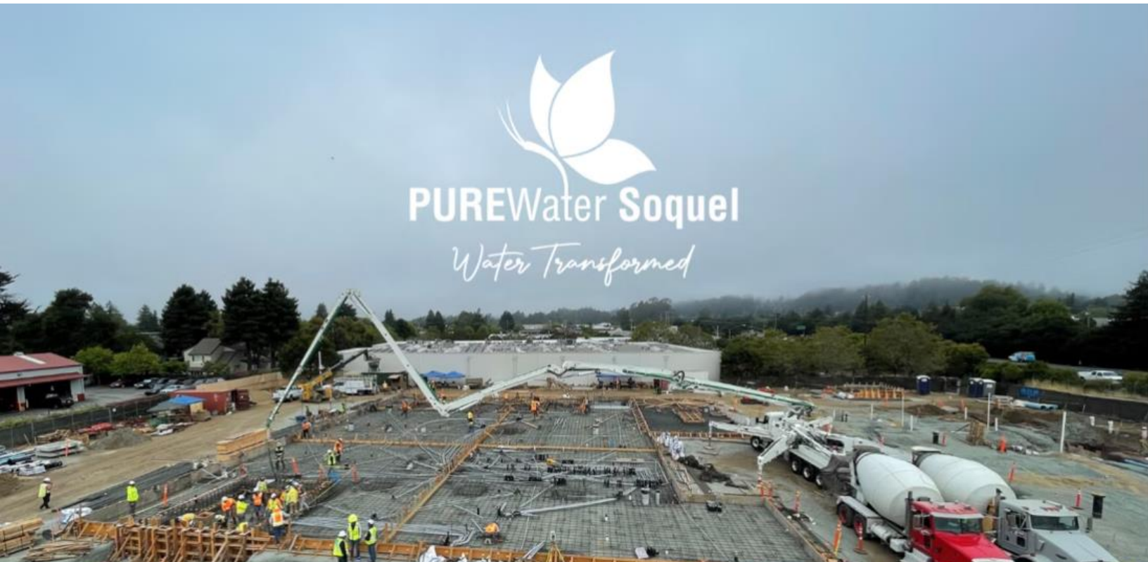
Figure 4-11: Pure Water Purification Center Construction
